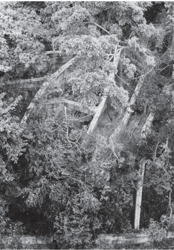
Figure 15. Reinforced concrete grid-beam system with wire netting infill
