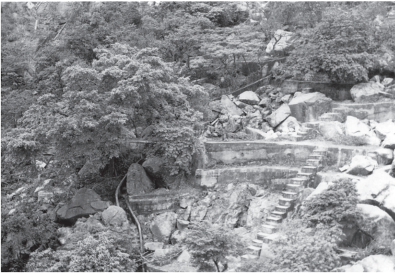
Figure 2. Concrete blanket in the form of terraces
