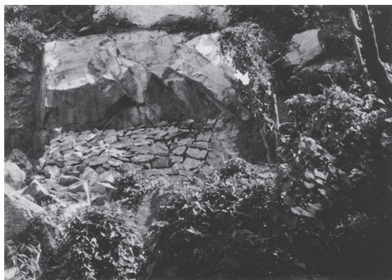
Figure 12. Masonry buttress
