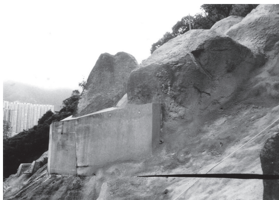
Figure 13. Mass concrete buttress (see also the surface protection)
