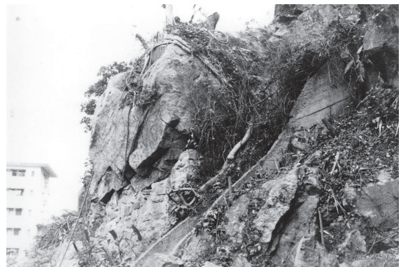
Figure 10(a). Splitting to remove overhang (before)
