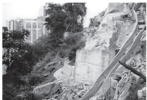
Figure 10(b). Splitting to remove overhang (after)
